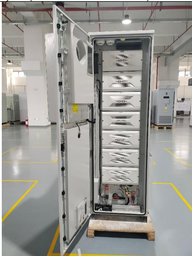
Opening view of battery system (Model: OLP-EB-V309 E63-AO01)
