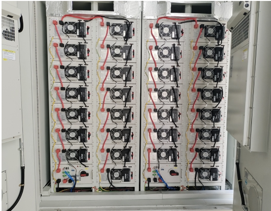
Photo 4 photo of the Battery cluster inside the Sample are not connected to each other. 图片 4 样品内电池簇相互不连接
